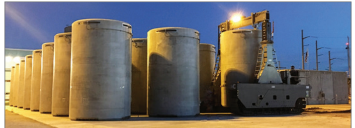
Top photo: Transport of 24th MAGNASTOR system to Kewaunee ISFSI pad. Bottom Photo: NAC MAGNASTOR spent fuel casks in storage at the Kewaunee ISFSI.
